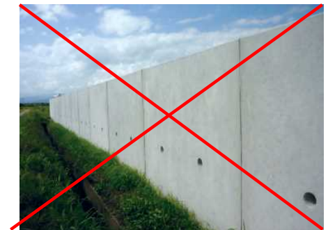
Oppressive vertical retaining wall of more than 2 m
